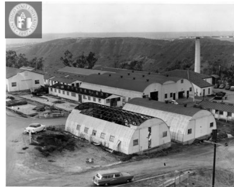
Figure 1. A photo of the temporary Engineering Buildings in 1959 [4].
