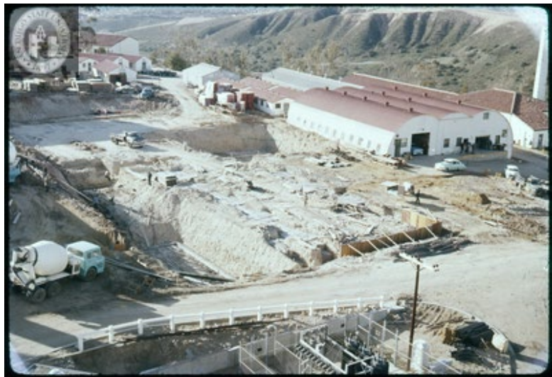
Figure 4. Construction of the engineering building in 1960 [17]. Note the basement floor to accommodate the low-speed wind tunnel being dug out in the left-foreground of the image.
